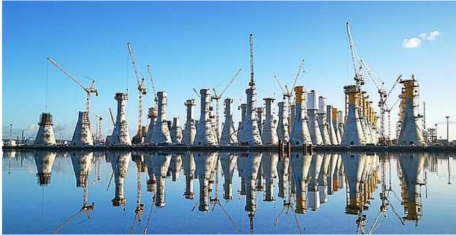
FIGURE 1 – Fécamp wind farm GBS under construction. Bouygues Travaux Publics. © Jacques Basile.
