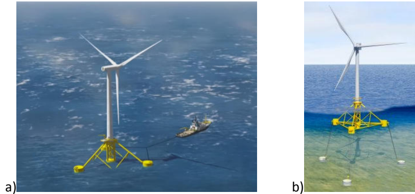
Figure 1-1: Artist views of the concept in a) towing and b) operational configurations
